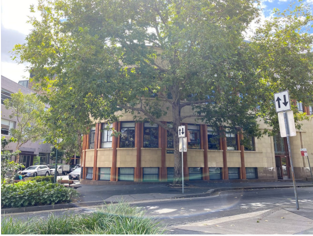
Figure 7: View of 80 Commonwealth Street 'Paramount Building' from Hunt Street
