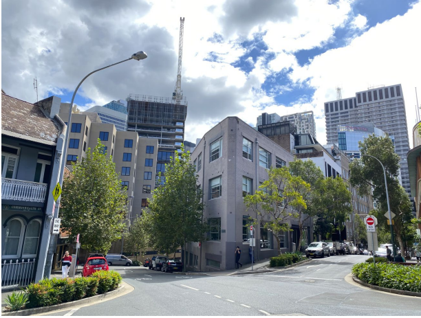
Figure 2: View of the site from intersection of Commonwealth, Hunt and Goulburn Streets
